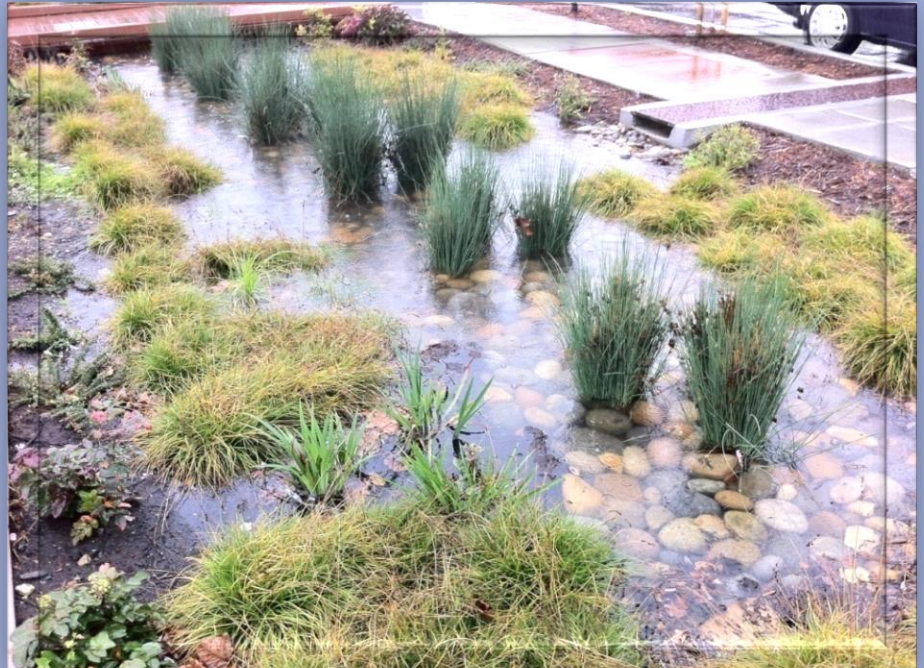
Donnelly Avenue Rain Garden, Burlingame
