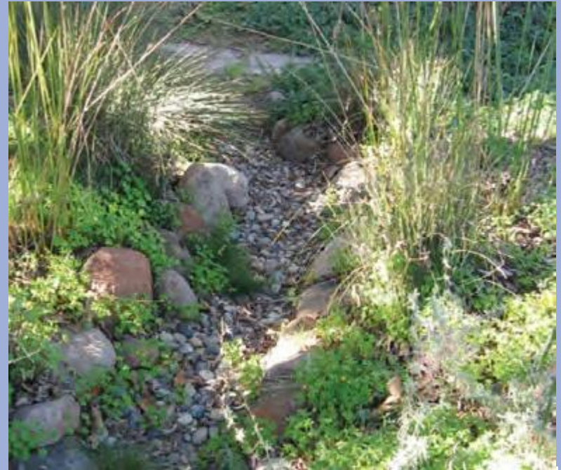
Dry creek infiltrates and conveys runoff.
